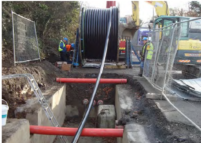
Typical HV Cable Installation
