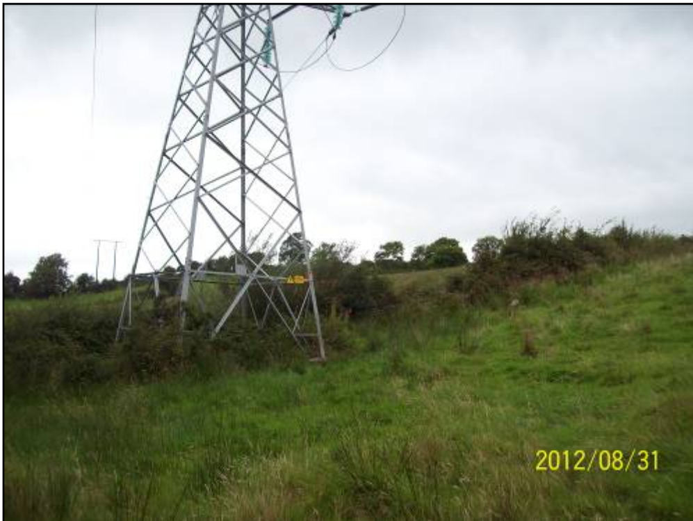
10L125 Ballyroe, Co. Clare 1km LHS Managed
