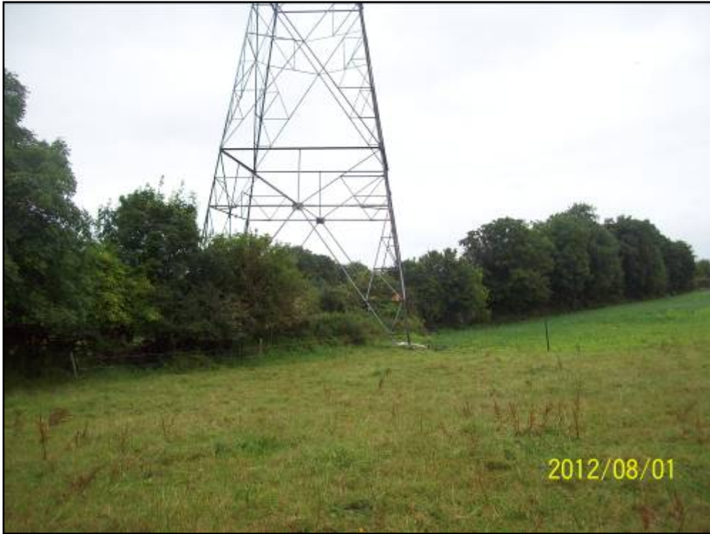
10L417 Knockatermin, Co. Clare 1km LHS Unmanaged
