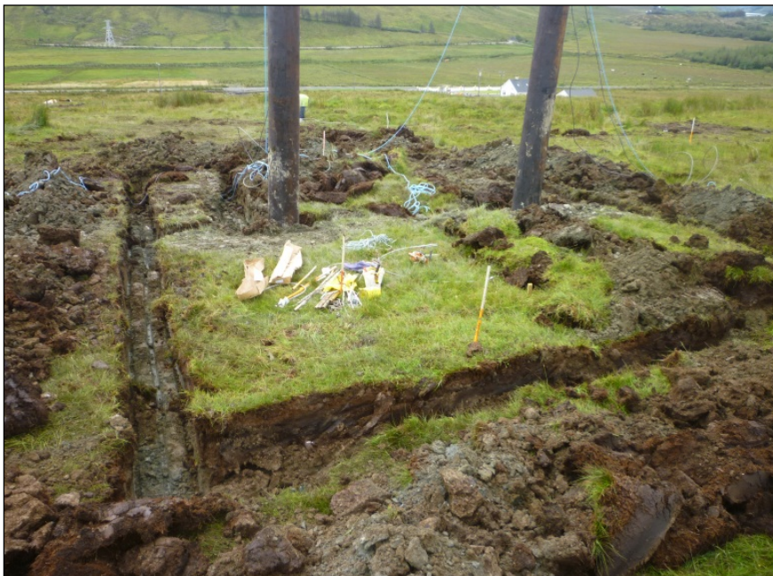
Earth ring on Donegal 110kV Project
